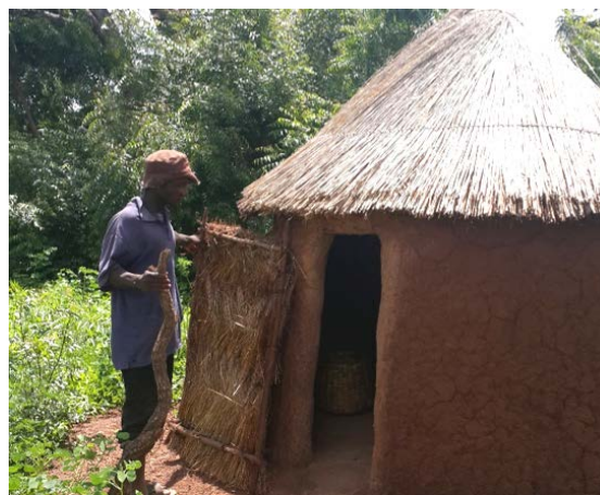
Members of Memunatu's family use this newly constructed household latrine.
