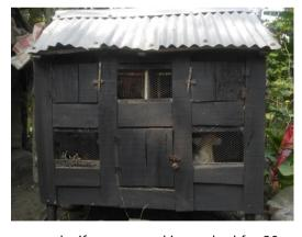
feet of space and there must be 0.5 square feet for every chick. For example, if you are making a shed for 20 chicks and 6–7 chickens, the house must be 4 feet long, 2.5 feet wide, and 3.5 feet high. A double-tiered house is preferable. The top of the shed can also be made with roofing grass or rice hay covered with polythene to protect it from monsoons.
